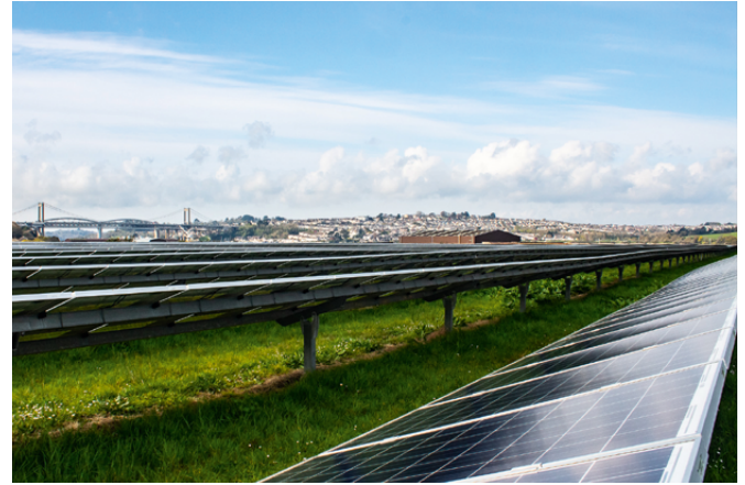
Solar farm in Plymouth, RegEnergy pilot project © Plymouth City Council
